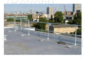
OSHA approved Perimeter warning and guardrail systems that is temporary and portable safety system that provides protection for workers and equipment from going into hazardous areas that may cause severe safety risks.
