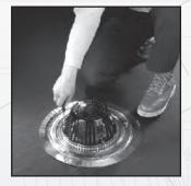
Upon completion of installation, feel and visually check the inside of the drain outlet to make sure it has been sufficiently expanded. Then, flash the flange to the membrane according to the instructions of the roofing system manufacturer. If clamping ring is used, hand tighten bolts using 7/16" (11mm) wrench. Secure strainer with the 3 bolts supplied.
